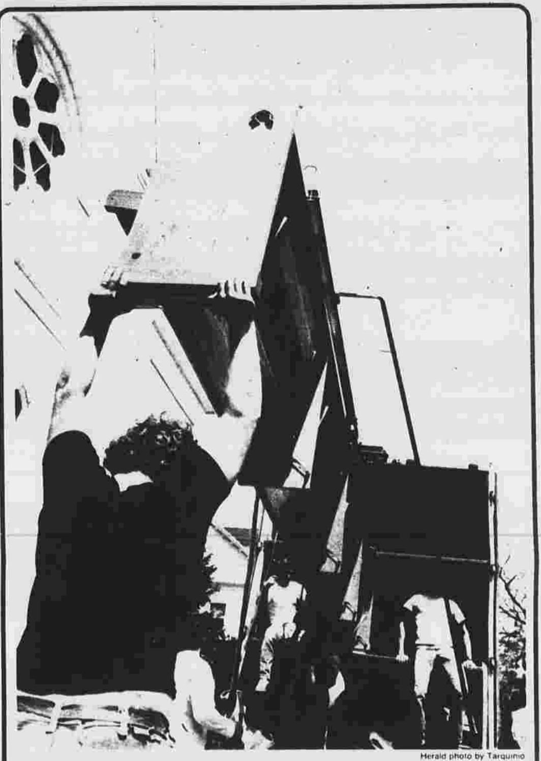
Workers from an Ohio-based company unload one of 50 new pews that have been installed at St. James Church this week as part of a major renovation project. The renovations, scheduled to be completed soon, were required to bring the 110-year-old Catholic church at 896 Main St. up to code, said Father Francis Krukowski.
